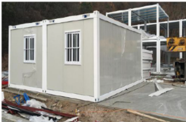
Figur 4.10 Konteiner-type prefabrikkert modul for isolat. Kilde: Luo et al. Foto: China Construction Third Engineering Bureau Co., Ltd
