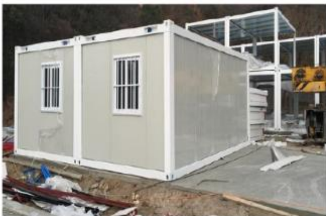
Figur 3.10 Konteiner-type prefabrikkert modul for isolat. Kilde: Luo et al. Foto: China Construction Third Engineering Bureau Co., Ltd
